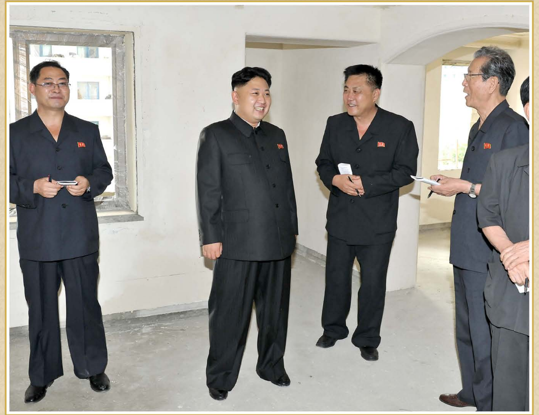
Kim Jong Un visits the construction site of apartment houses for scientists of Kim Il Sung University in August Juche 102 (2013).
