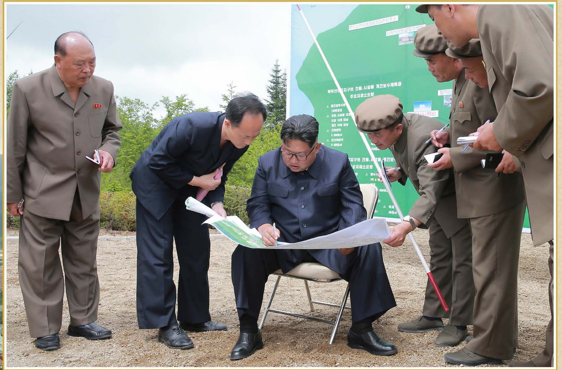
Kim Jong Un gives on-site guidance at construction sites in Samjiyon County in July Juche 107 (2018).
