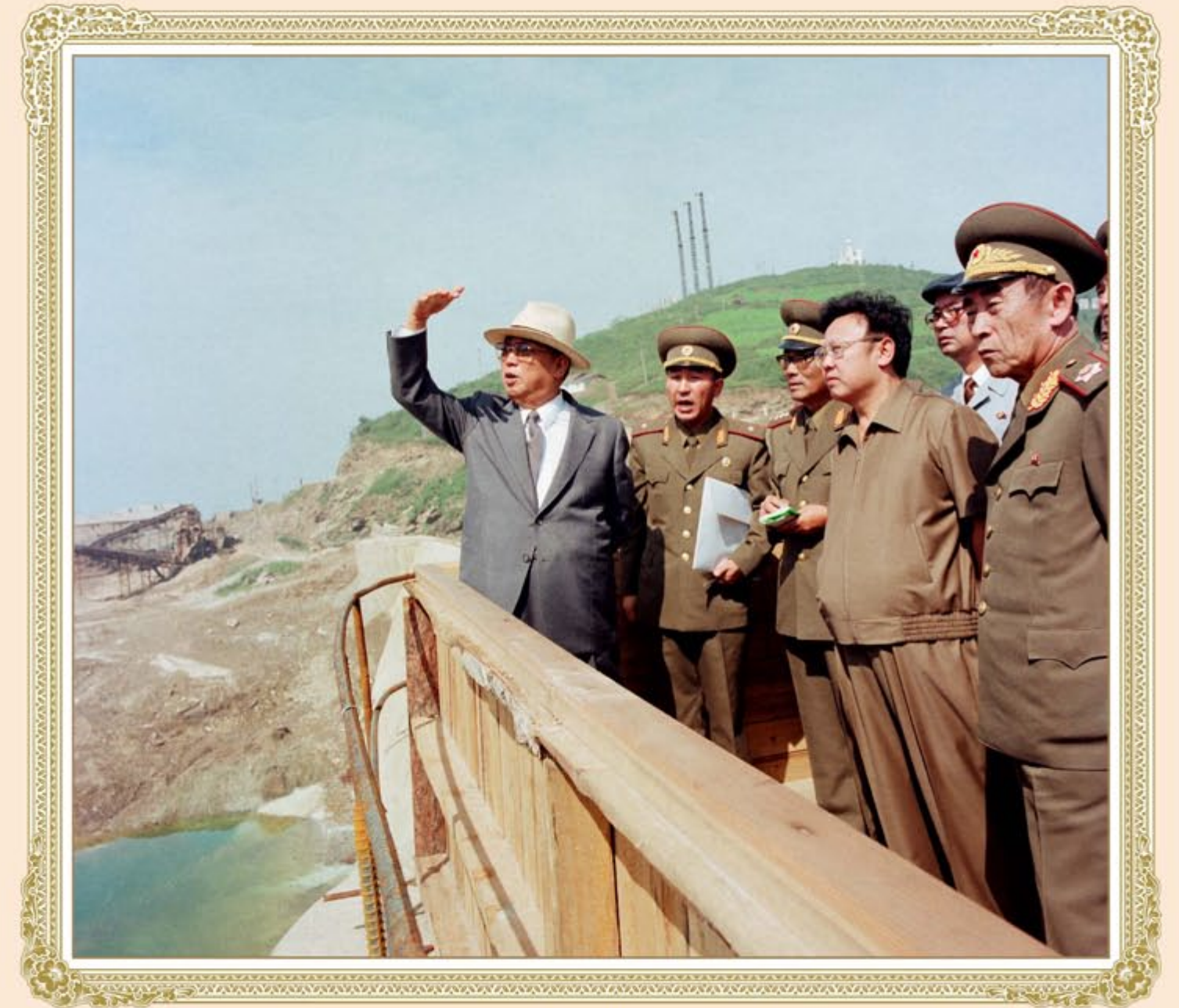
Kim Il Sung and Kim Jong Il giving field guidance at the construction site of the West Sea Barrage in September 1985
